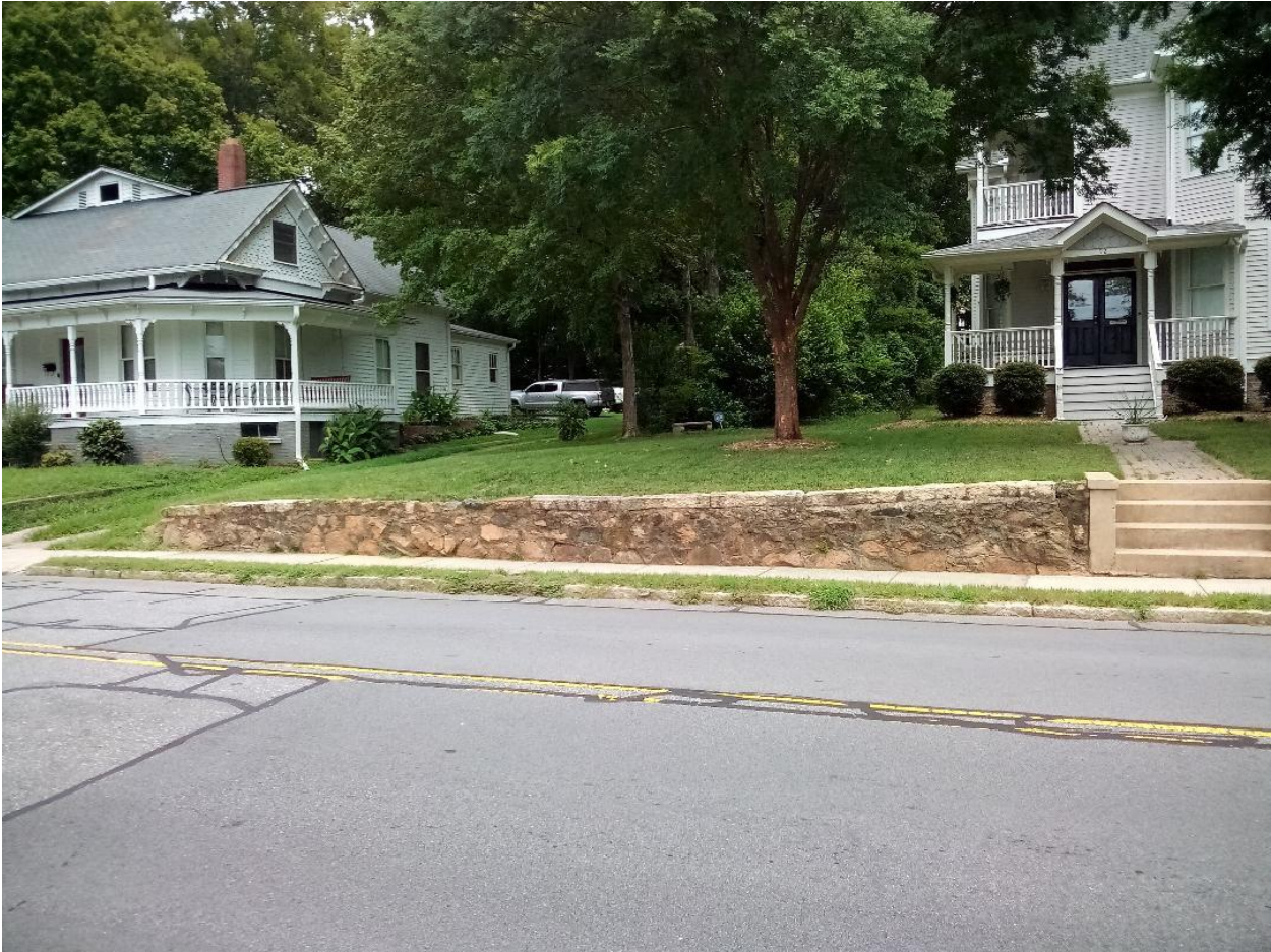
H-19-22 Existing Masonry Retaining Wall – Left Side
