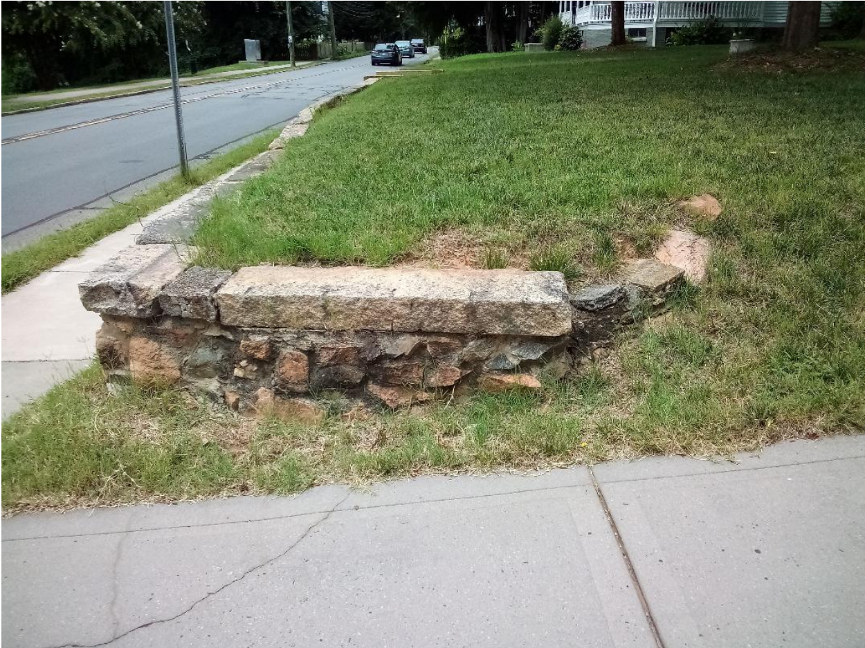
H-19-22 Existing Masonry Retaining Wall – Front to Back Along Driveway Entrance
